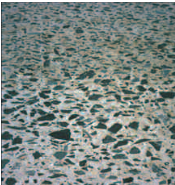
Figure 72: Distress Type JCP 9 Polished Aggregate
