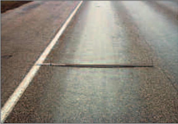
Figure 32: Distress Type ACP 9 - Rutting
